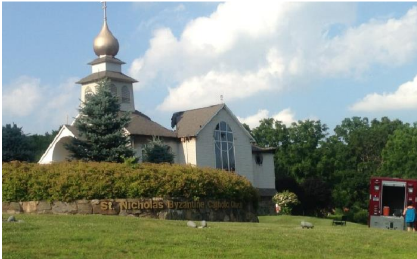
St. Nicholas Church, a landmark on Pembroke Road in Danbury, is heavily damaged after a fire Saturday. The roof behind the onion dome has collapsed. Photo Credit: Karen Tensa
